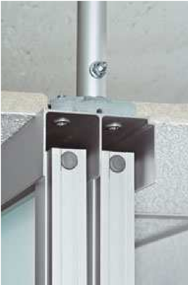
The installation of the top track using a track connector.
