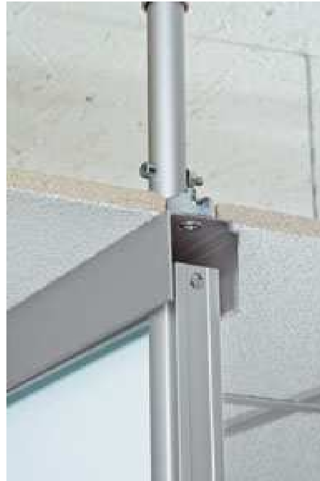
The installation of the top track using a track connector.
